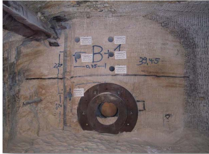
Figure 5. Photograph of the BAMBUS II re-excavation.
